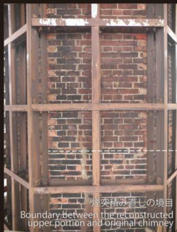
煙突内部の段差 Inner corbelling of the present chimney
