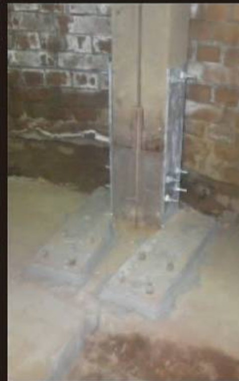
柱足元の補強 Reinforced column end
