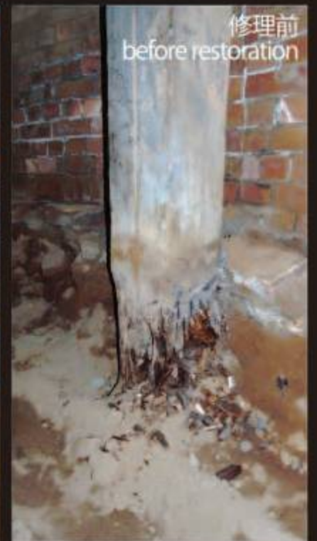
修理前 before restoration 掘立て Buried column end
