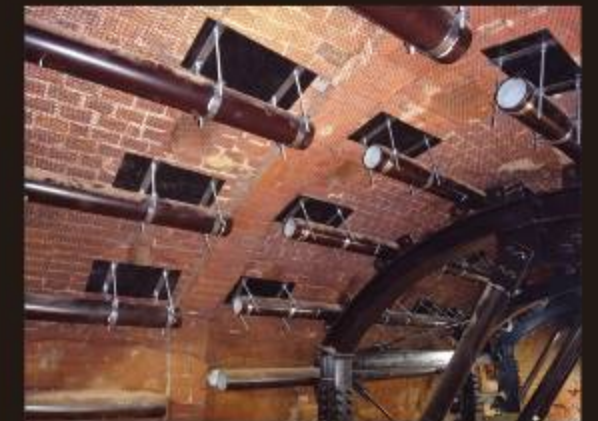
見える補強の鉄骨 Steel frame as visible reinforcement
