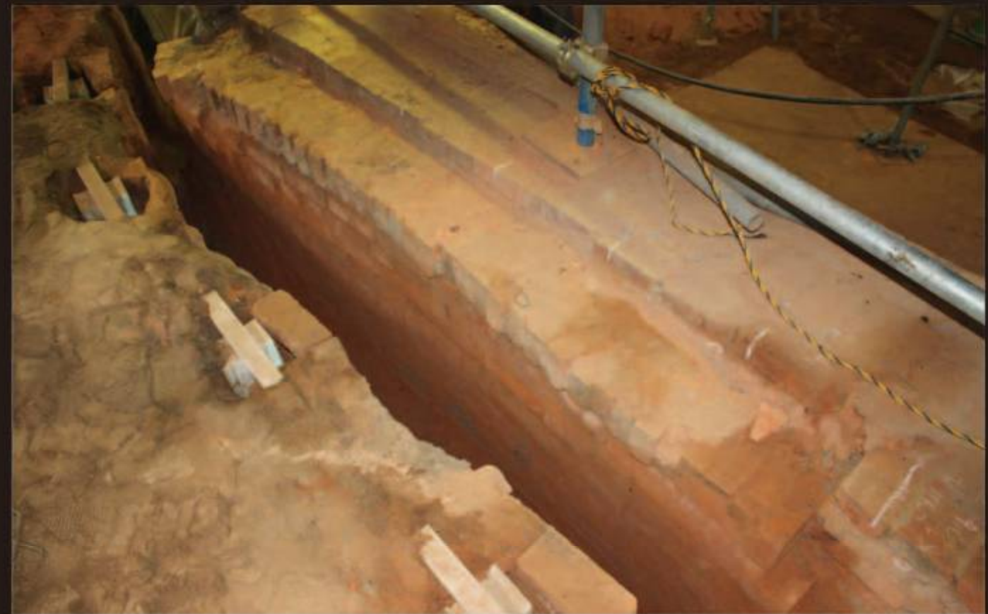
9号窯で確認された旧土留壁 Retaining wall discovered near chamber 9
